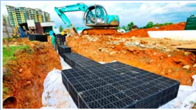
VersiTank® Infiltration System installed at a park
